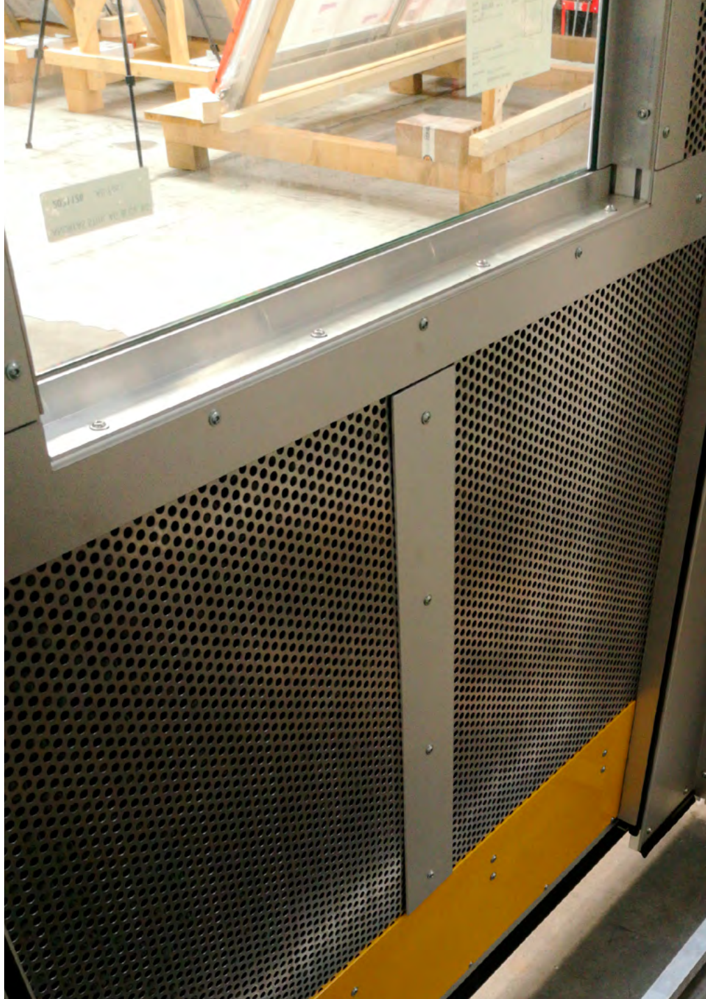
Sound insulation by means of terodem panels and perforated metal sheet (rear view)
